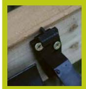
If you do not use longer screws - as the Alpaca naturally push down onto the drainpipes when feeding, the short screws will come out and the drainpipe will flap and fall.
